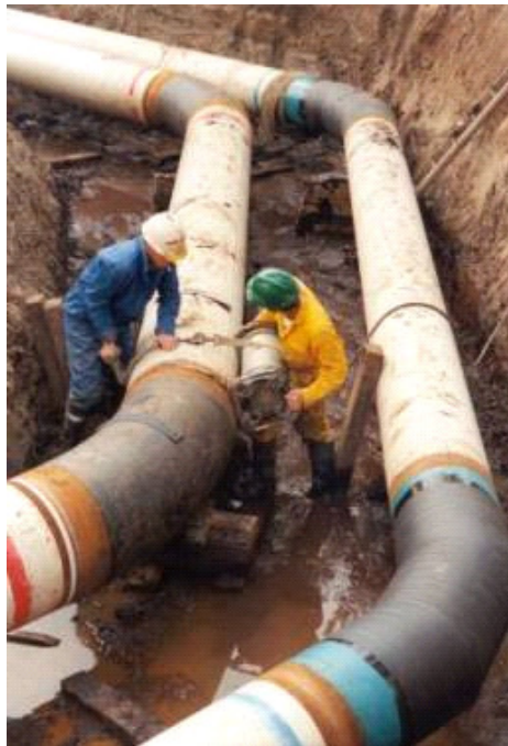
Figure 8. New, large diameter pipelines are expanding
