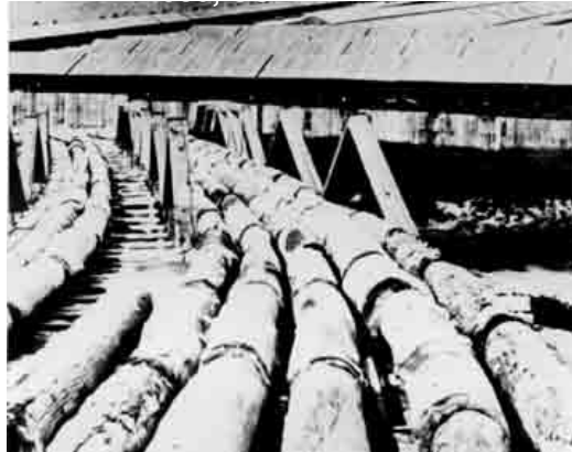
Figure 2. Hollowed-out logs used to transport brine circa 1880
