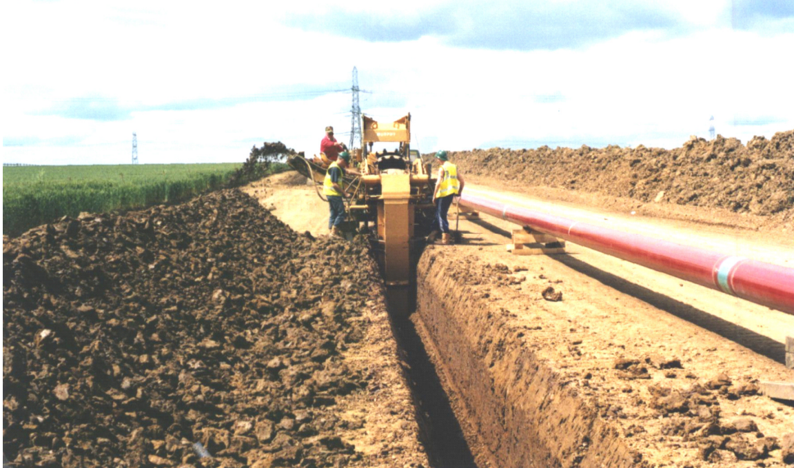
Figure 10. Pipelines are critical transportation infrastructures
