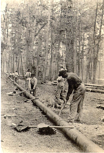
Figure 7. Early pipelines were joined and laid 'by hand'
