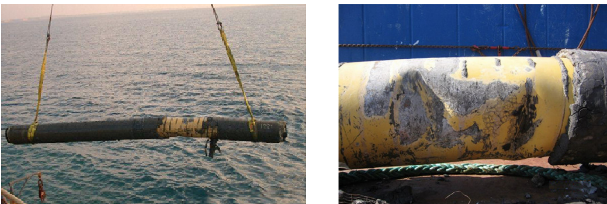
Figure 7. Damage to a subsea pipeline [30]
