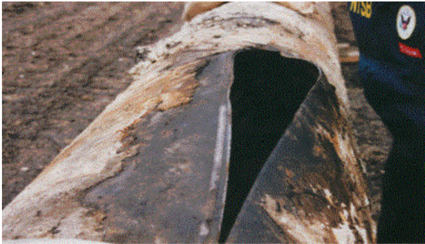
Figure 7. Rupture along defective seam weld (taken from The National Transportation Safety Board website: www.nts.gov ).
