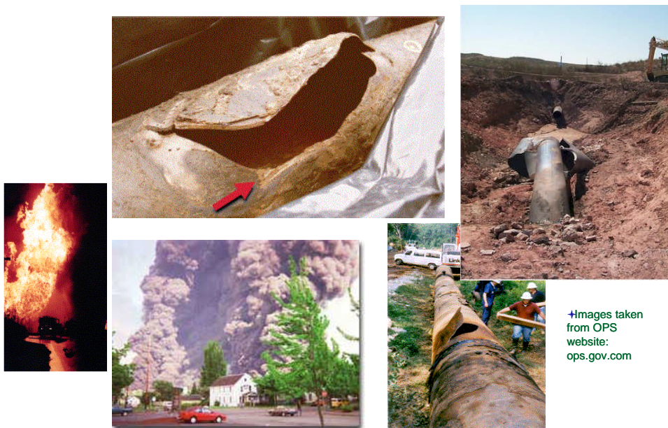
Figure 1. Recent failures of pipelines in the USA [4] (images courtesy of the Office of Pipeline Safety, USA).
